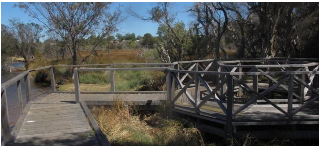
Plate 1 Boardwalk at eastern end of Baigup Wetland Reserve
