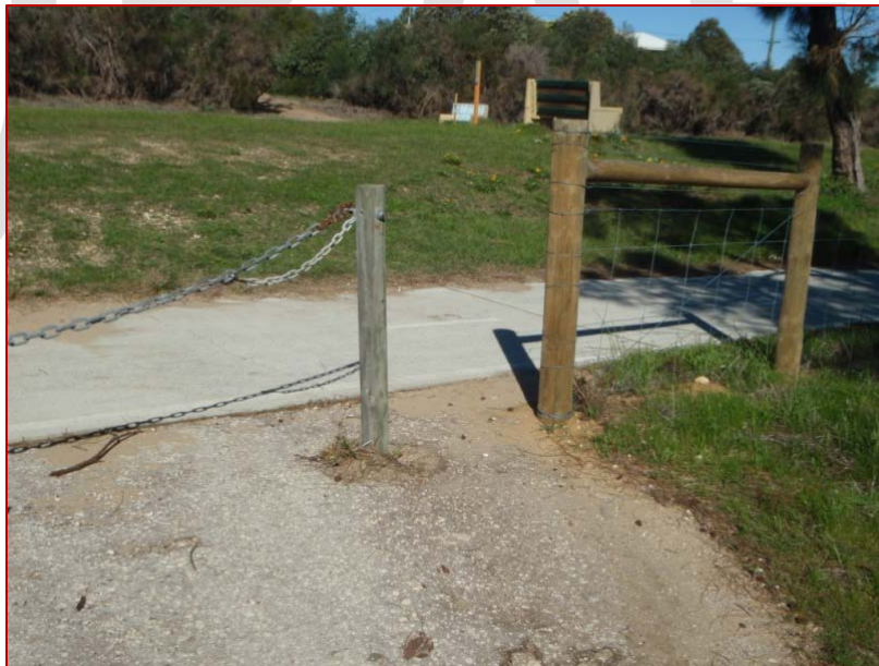
Figure 37: Typical Pedestrian Access Point next to a Vehicle Chain Gate
