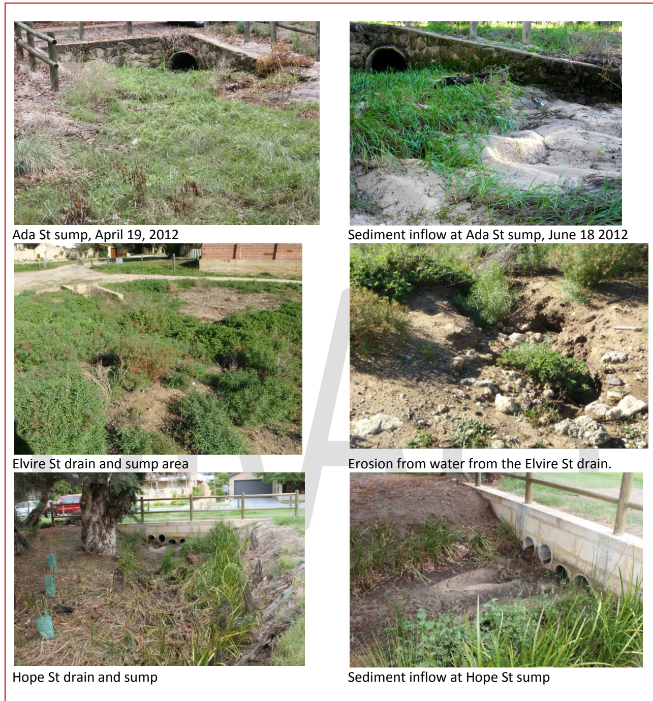
Figure 7: Drains and Associated Sumps Entering Star Swamp
