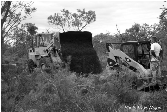
Bringing in topsoil on track to Roe Highway.
