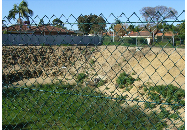
An example of a typical sump where herbicides are used to control weeds.
