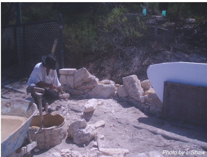
Photo by L Shaw One of the stonemasons in action building the limestone rubble wall at the entrance to Allen Park Bushland.
