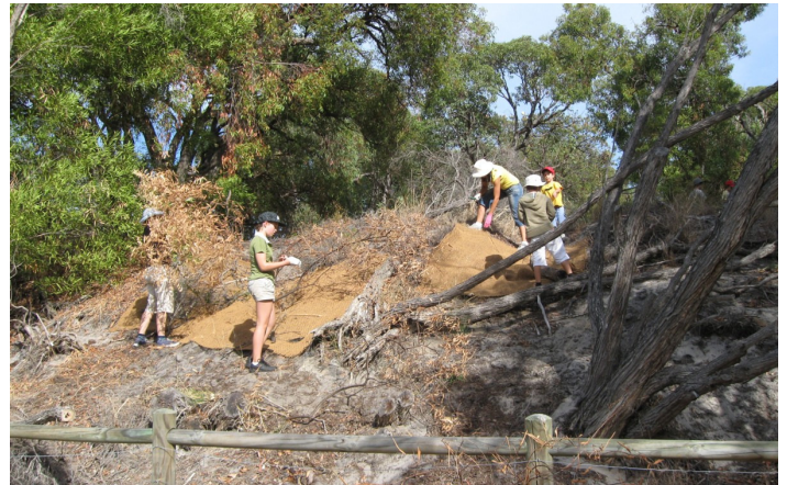
Friends of Coolbinia Bushland stabilizing an eroding embankment.
