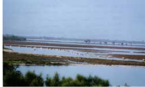
Separation canal flooding the wetland
