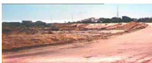
Work on Area A
