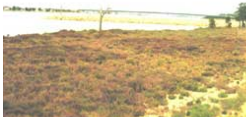
Samphire at Entrance Canal. Note new wall out into estuary
