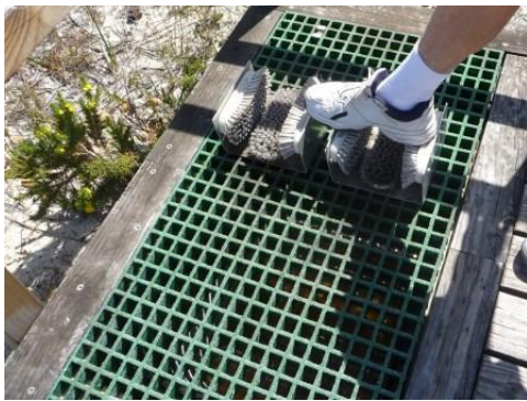
Figure 11: Grated shoe cleaning station to prevent spread from dislodged material. Photo: State NRMWA
