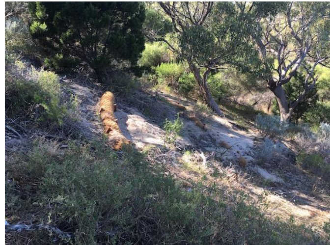
Erosion control - coir matting installation
