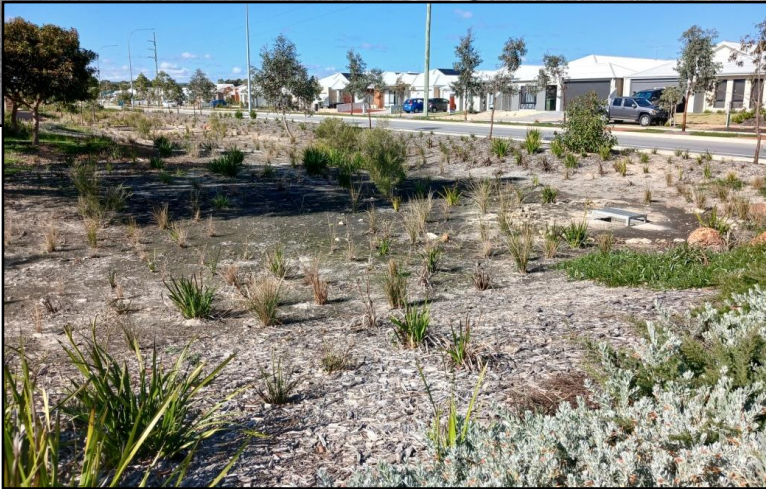
Swales and bioretention basins to Woolcott Ave, Brabham (above) and Queensbury Drv, Dayton (right) are a portion of hundreds of kilometers Water Sensitive Design devices in new urban
